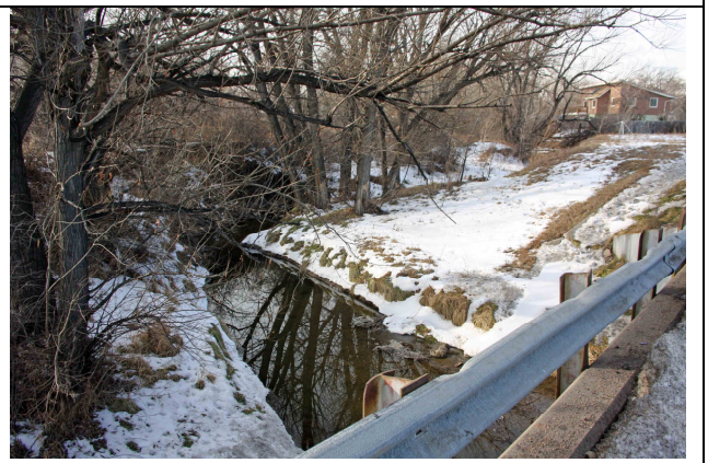
Figure 6. View looking southwest at a southern tributary of Lakewood Gulch on the south side of 6 th Avenue west of Wadsworth Boulevard.
